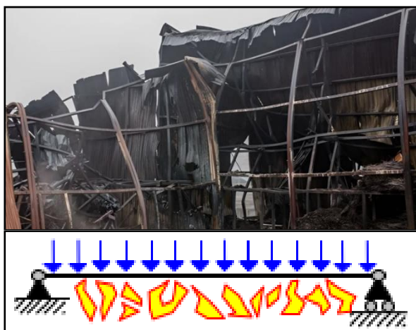
Figure 3 – Appearance of metal frame after a fire and design sketch of the beam by fire effect
