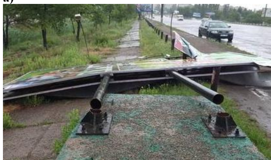
Figure 1 – Advertising structures that did not withstand the load (a, b).
